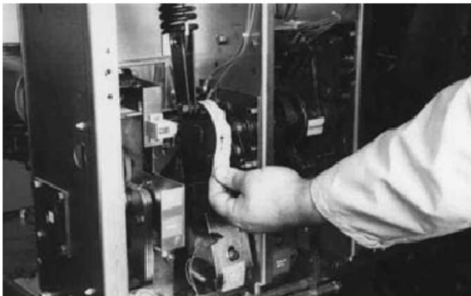
Figure 6-16 Remove Marked Masking Tape From Cam
