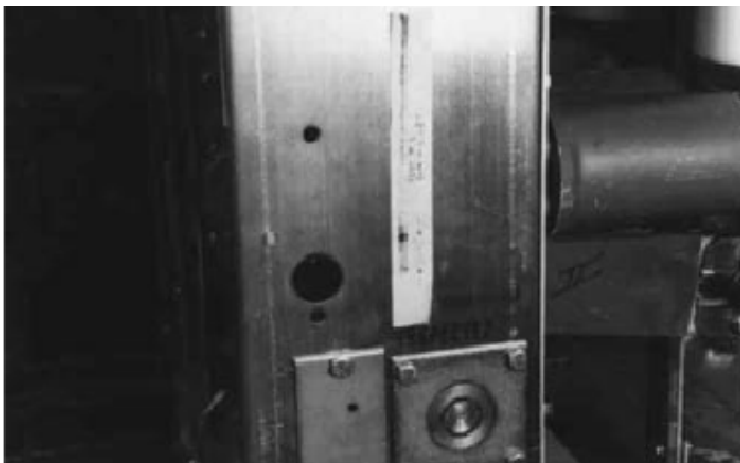
Figure 6-17 Place Tape On Right Side Panel of Breaker
