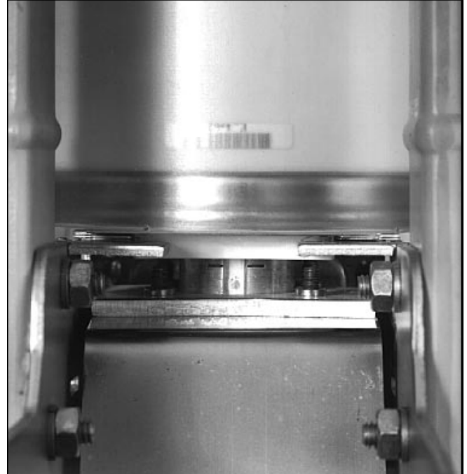
Figure 6-3 Vacuum Interrupter Showing Contact Erosion Indicator with Breaker Closed (Indicators are Checked Only When Breaker is Closed)
