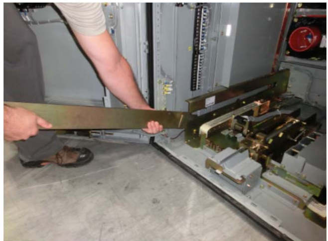
Figure 4-2A Insertion of the Drawout Extension Rails
