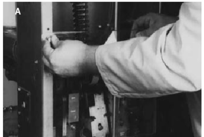
Figure 6-9 Attaching CloSure™ Test Tool at Hole “A”
