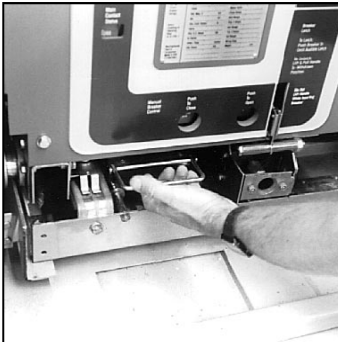
Figure 4-5 Pulling Secondary Disconnect Cage to Engage Secondaries in TEST Position (Old Version Shown). New Version will have BPI Pan With Automatic Secondaries.
