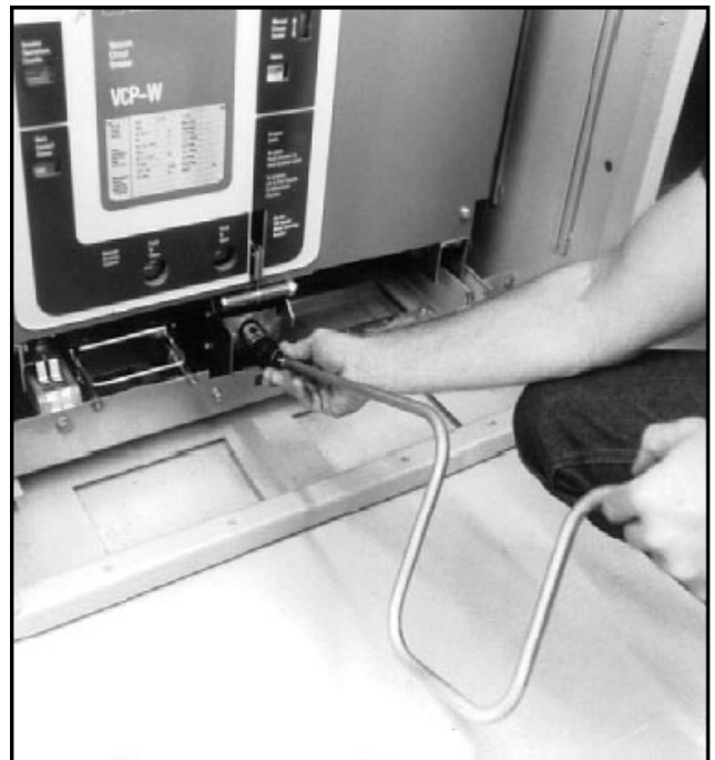
Figure 4-6 Engaging Levering-In Crank
